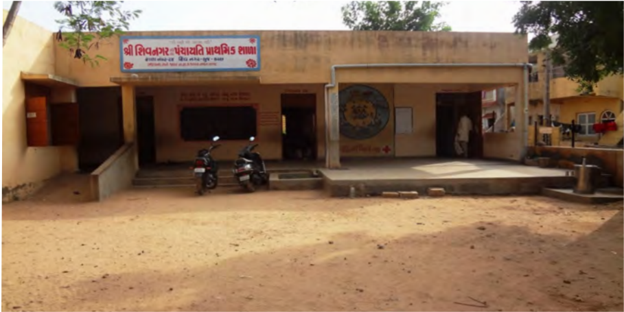
A groundwater recharge pit at Jubilee Colony (top) and an installed RRWH system in a government-run primary school at Shivnagar (bottom)
