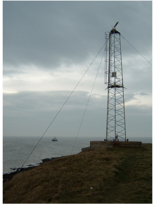
Fig. 1. A photo of the radar tower looking north on Hilbre Island.
