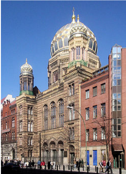
The restored Neue synagogue in Berlin
