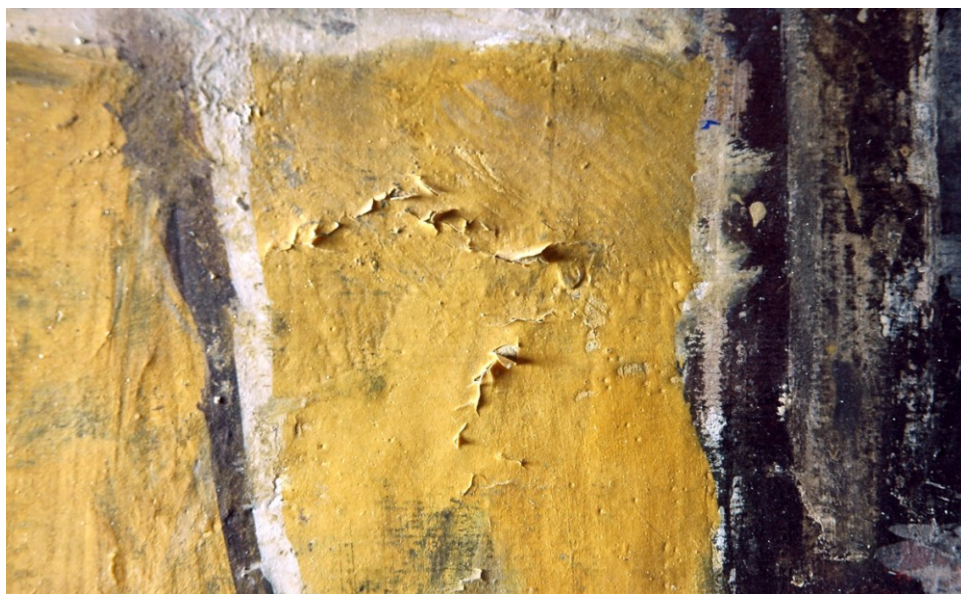
Fig 46 Detail in raking light of a detachment of the pictorial layer.
