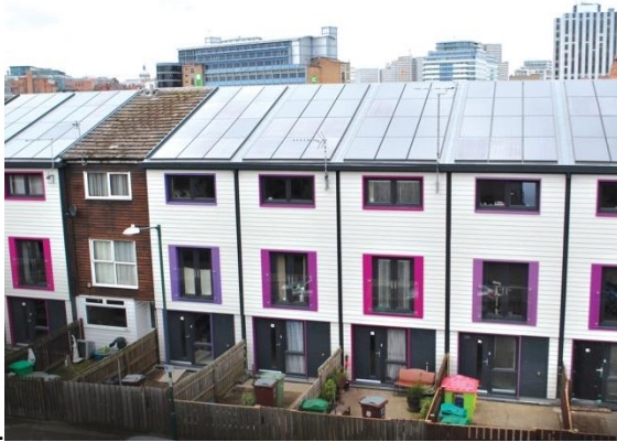
Figure 3.2 Energiesprong Nottingham retrofit
