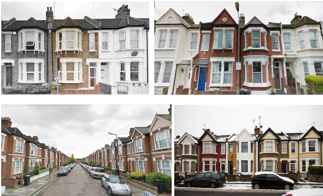
Figure 4.8 Examples of Terrace houses with bay windows Clock wise, a, b and c photos taken by the researcher, d, Brent, London, RfF programme project (Image credit: Low Energy Building Database, www.lowenergybuildings.org.uk )
