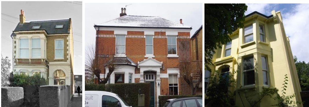
Figure 4.5 Examples of Detached houses Left to right, a and b photos taken by the researcher, c, The Nook, Lover's Lane, Brighton, RfF programme (Image credit: Low Energy Building Database, www.lowenergybuildings.org.uk )
