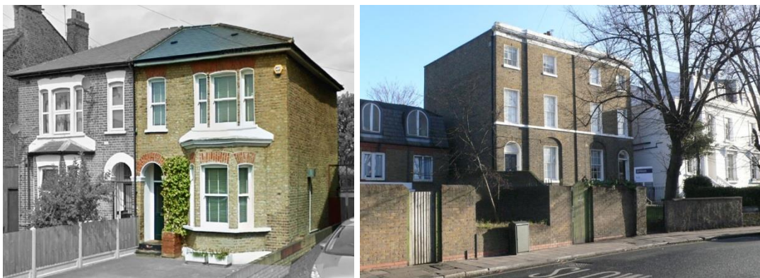
Figure 4.6 Examples of Semi-Detached elevations Left photo by the researcher, right Clapham Retrofit, Arboreal Architecture (Image credit: Low Energy Building Database, www.lowenergybuildings.org.uk )
