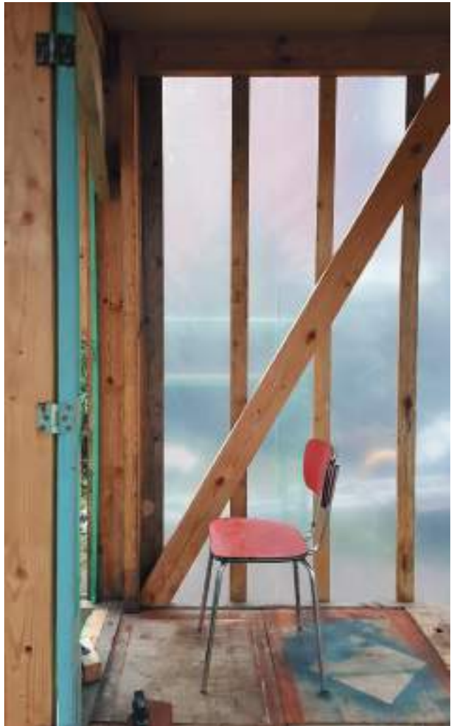
00.04.fig.20 – The Maison des Possibles at Josaphat, under construction, December 2017.
