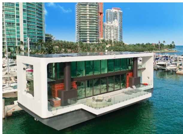
Fig. 36 Floating house by Arkup.
