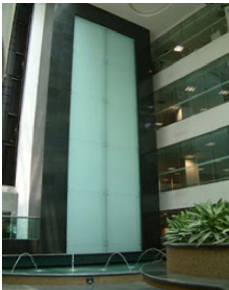
Fig. 33 Water wall for cooling strategy in the atrium of LEO Building in Putrajaya, Malaysia.
