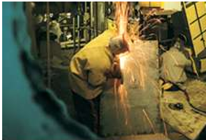
Fig. 1. Nuclear decommissioning worker wearing an air-fed plastic suit underneath a heavy leather overcoat, and multiple layers of gloves, while using power tools to cut legacy nuclear plant contaminated by alpha-radiation emitting substances, such as plutonium dust. The leather coat protects the plastic suit from being punctured by hot sparks during cutting. Maximum 2hrs work per day is possible, due to extreme discomfort and heat exhaustion as the suit fogs and fills with sweat. Image courtesy of Sellafield Ltd.
