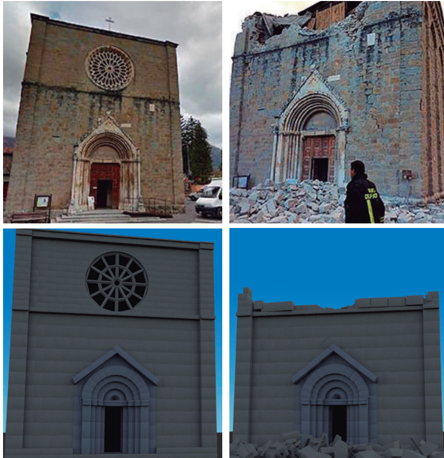
Figure 4.7: On the top, pictures from real St. Agostino church [27] before and after the earthquake took place. Below, the modelled church before and after the simulation of an earthquake with the similar properties as the real one.
