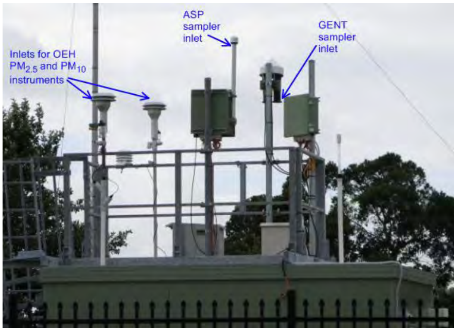
Figure 12 Identification of ASP, GENT and OEH inlets on the roof of the OEH Newcastle Air Quality Monitoring Station
