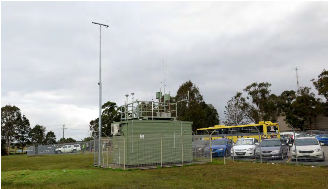
Figure 15 Beresfield Air Quality Monitoring Station located adjacent to Francis Greenway High School
