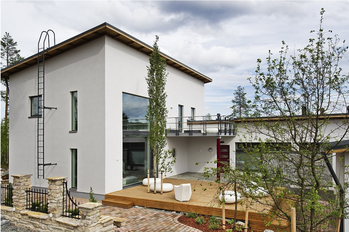
Figure 8. House A viewed from west
