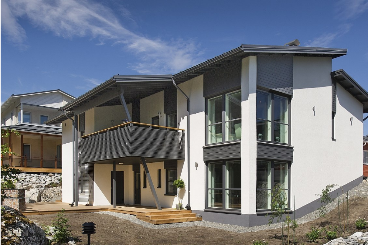
Figure 9. House B from southeast
