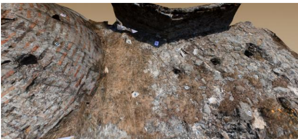
Figure 20. Detailed part of North West in superstructure
