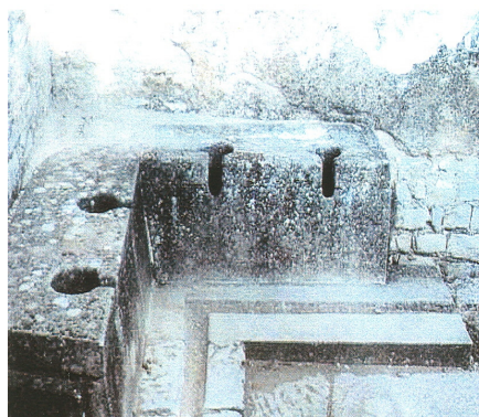
Figure 2.17. Public toilet, Latrine (Gülbay, 2003)
