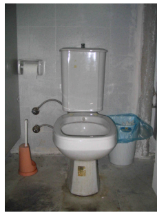
Figure 5.1. General view of a toilet stall
