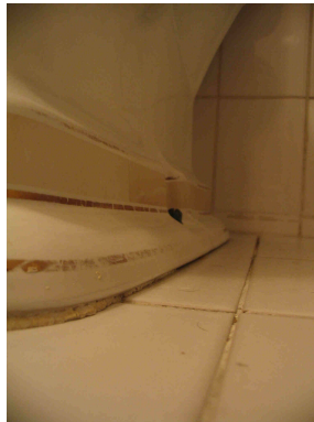
Figure 5.3. A toilet base
