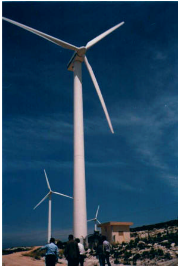
Figure 2.6 Horizontal axis wind turbines installed in Alacati/Turkey.
