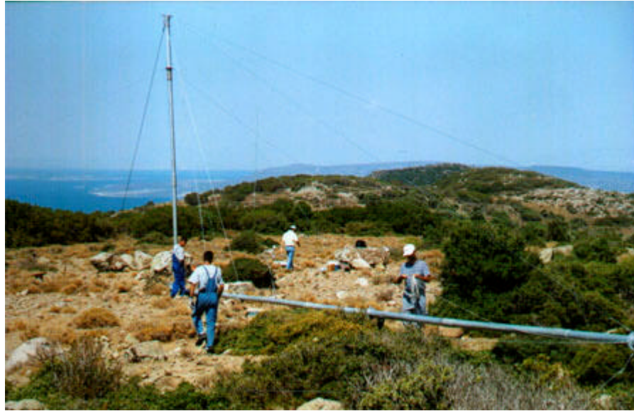
Figure 4.7 Erection of the IYTE mast.
