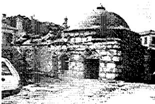
Figure 1. General view of the bath from the east elevation.
