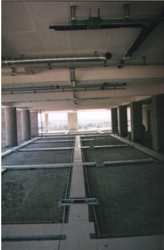
Fig. 4.25. Channel System Grid for Cabling
