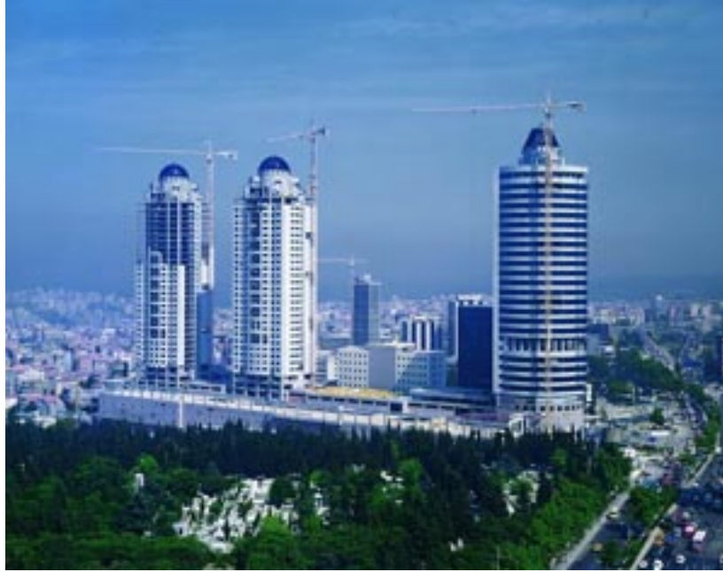
Fig. 4.1. Metrocity Millennium Towers Construction Phase (Source: http://www.hurriyetim.com )
