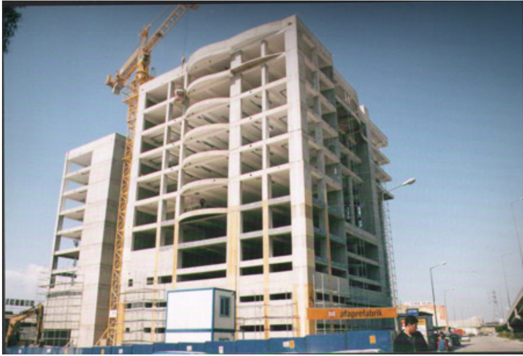
Fig. 4.21. Arkas Holding Construction Phase
