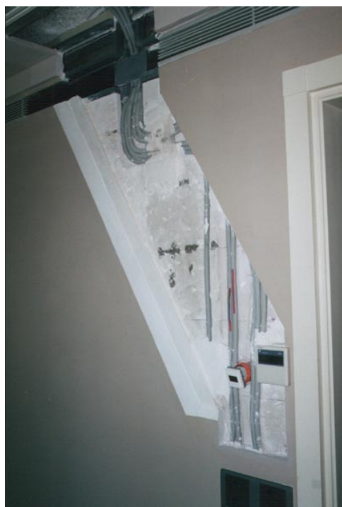
Fig. 4.5. HVAC Installations, Pipes and Connections to the Electronic Devices Hidden in Wall and Suspended Ceiling.
