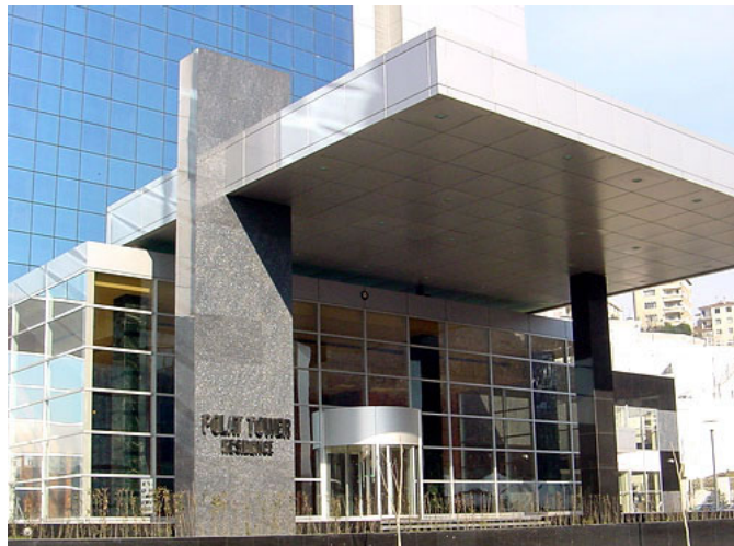
Fig. 4.8. Entrance and the Canopy of the Polat Tower Residence (Source: http://www.polatinsaat.com )
