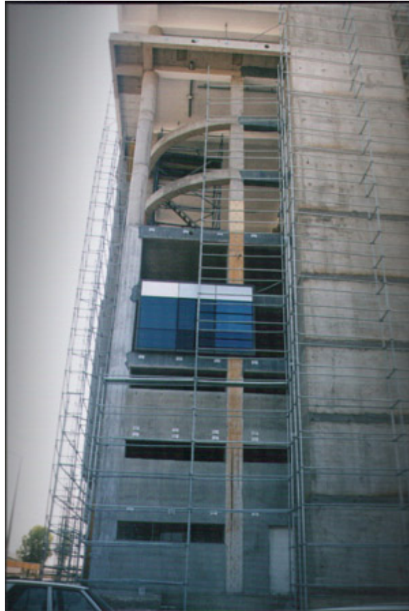
Fig. 4.23. Curtain Wall System of the Building
