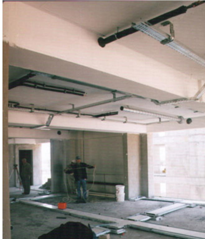
Fig. 4.27. Channel System Grid and HVAC System Construction
