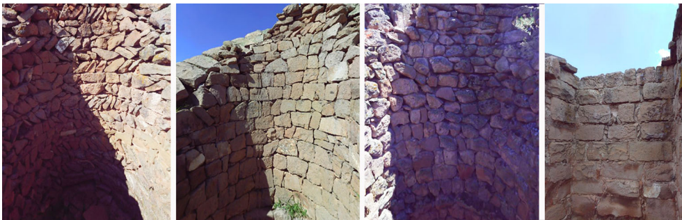
Figure 13. The inner stone masonry leaf: rough-cut masonry and cut stone masonry
