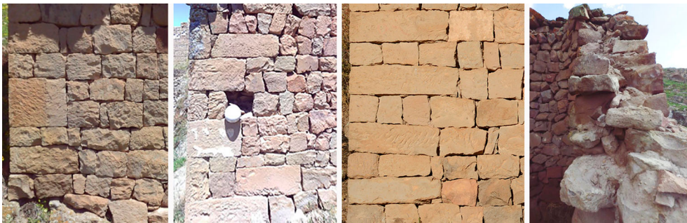
Figure 12. The outer stone masonry leaf: Different applications for the edges of tower and a wall with double-leaf.
