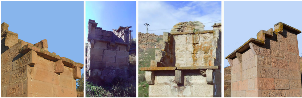
Figure 17. Eaves in the dovescotes built with cut-stone masonry: different applications.
