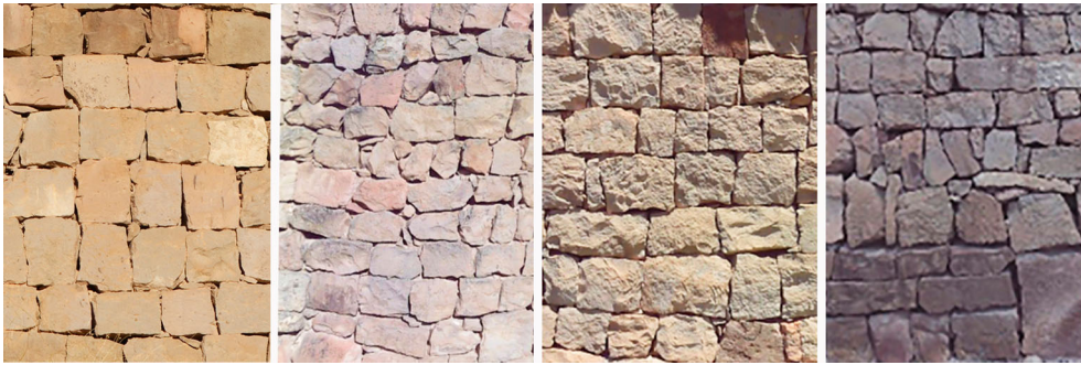
Figure 11. Use of stone in the outer leaf of the walls.
