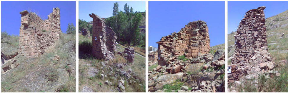
Figure 18. Damaged dovecotes in the valley.
