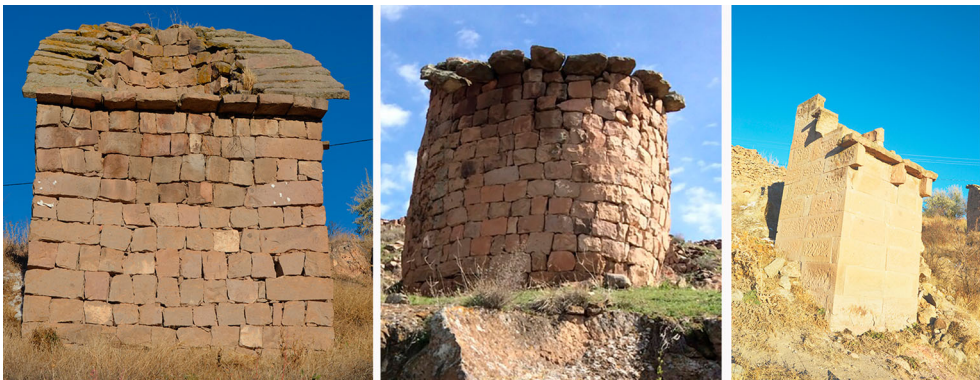
Figure 8. Examples for the towers of dovescotes in Kayabağ: U shape plan, circular plan and rectilinear plan.
