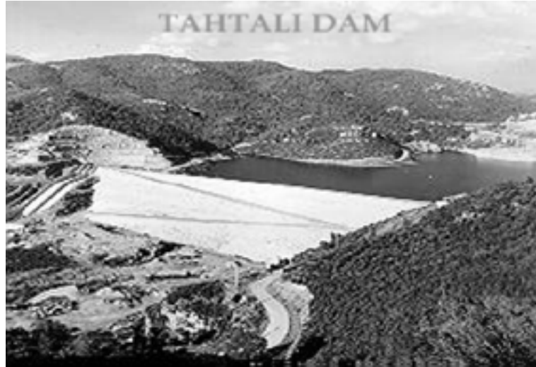
Figure C.1. General View Of Tahtalı Dam
