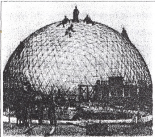
Figure 6.6 Framework for the Zeiss Dome.
