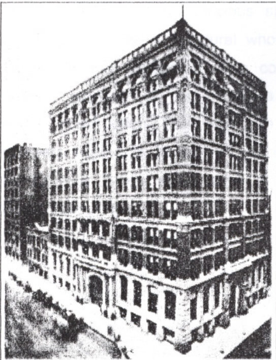
Figure 5.7. Home Insurance Building
