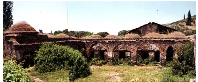
Fig. 4. Local construction technique composed of rubble stone, brick and mortar in random bond of Birgi Derviş Ağa Madrasa.
