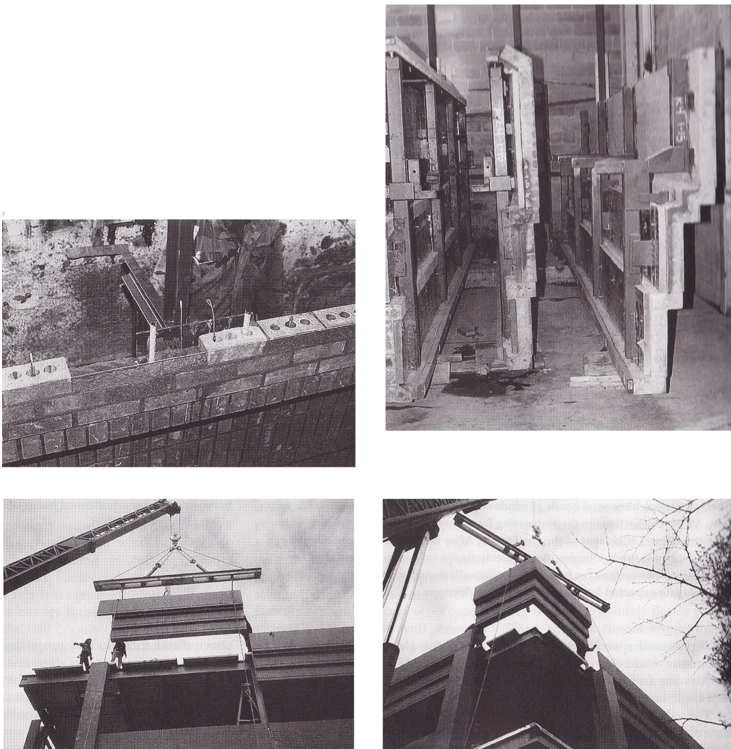
Figure 2.24. Fabrication and insulation of a brick panel curtain wall (Source: Allen 2004)
