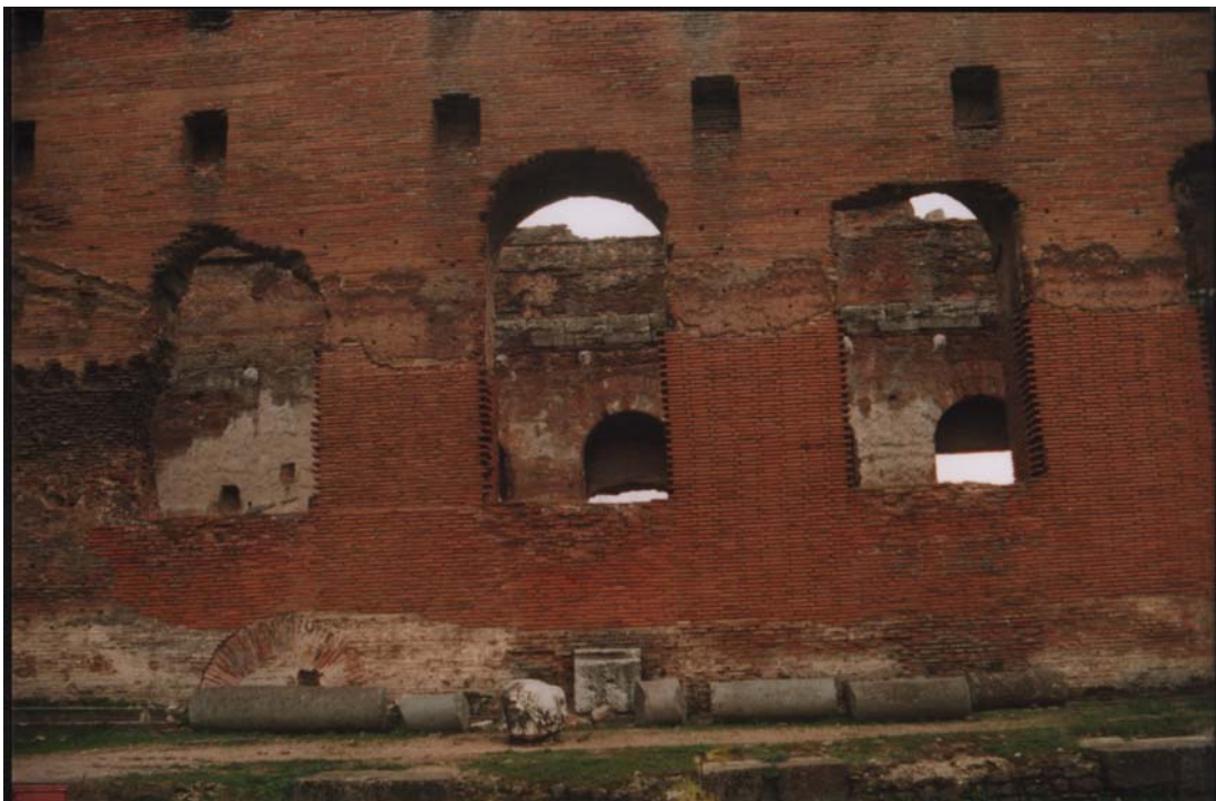
Figure 2. 13. A view of the north-east elevation of the restoration sections of the structure carried out in 1940s in the Serapis Temple (2004).
