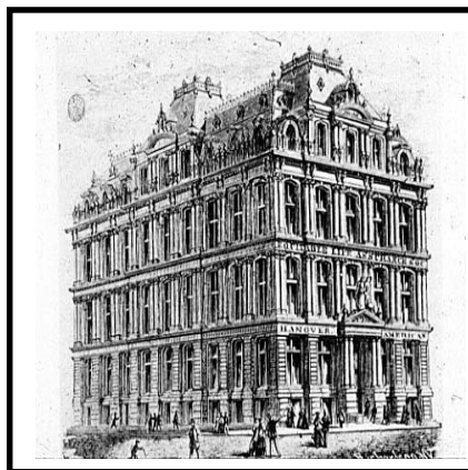
Figure 2.1 Equitable Life Assurance Building, 1868-1870
