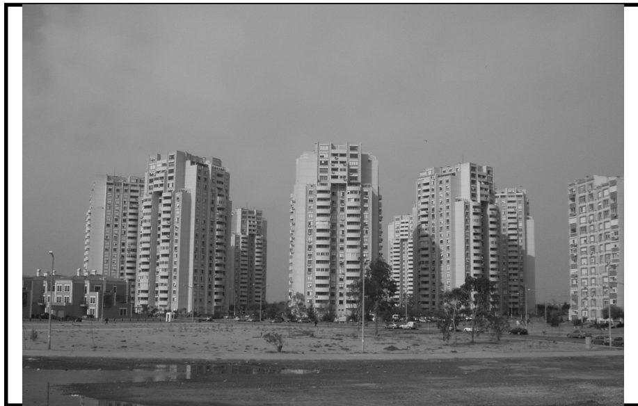
Figure 4.13. Mavişehir II; View of Albatros Apartment Buildings
