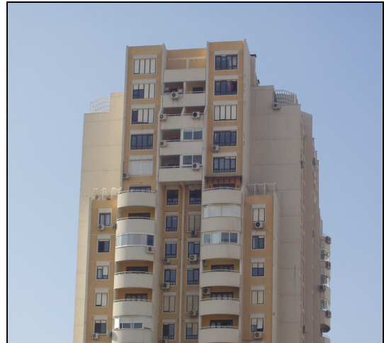
Figure 7.9. External View of Albatros Apartment Building
