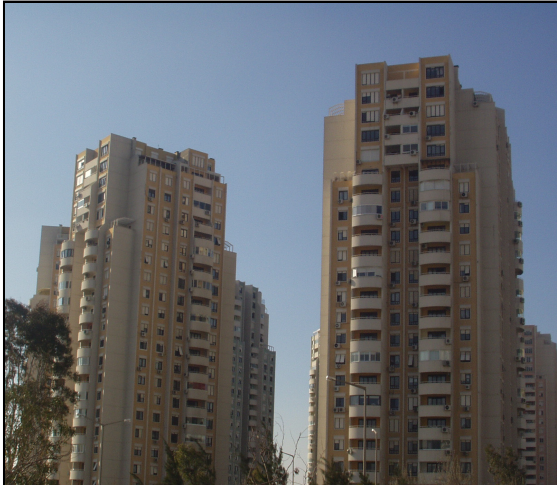
Figure 7.8. External View of Albatros Apartment Building
