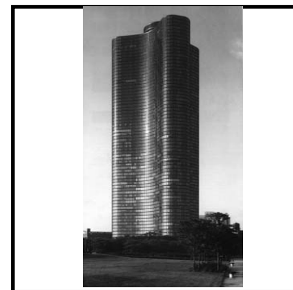
Figure 2.27 Lake Point Tower, 1968
