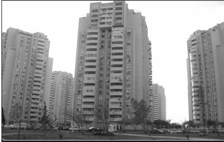
Figure 4.12 Mavişehir II; View of Albatros Apartment Buildings
