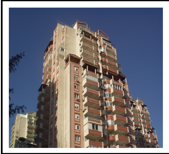
Figure 7.12. External View of Flamingo Apartment Building
