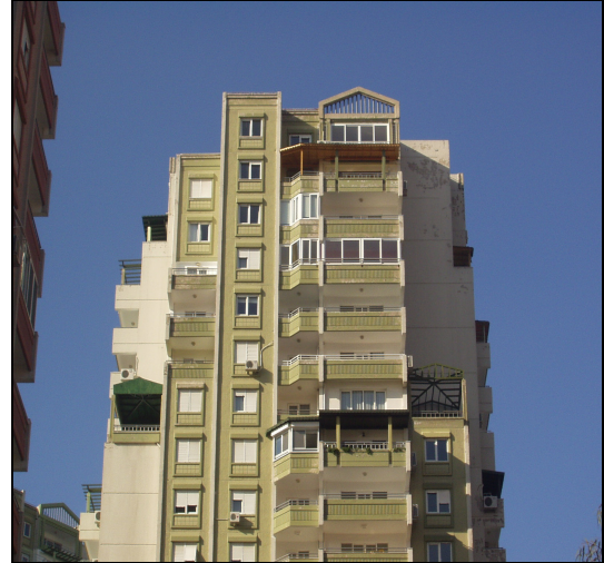
Figure 7.13. View of Flamingo Apartment Building
