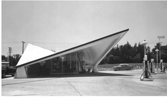
Figure 1 Hypar concrete shell.
