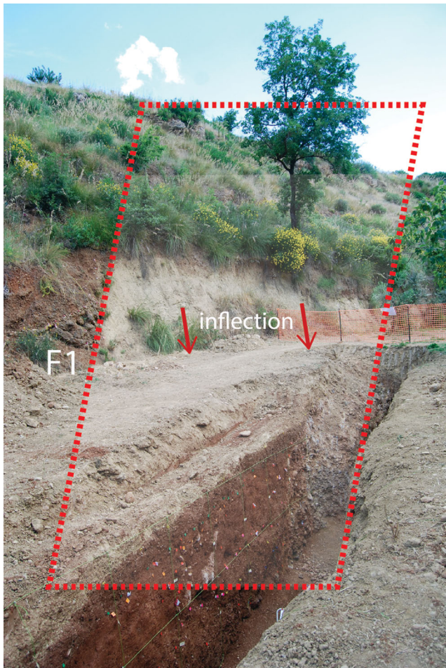
Figure 11. View of the excavation about 6 m from the northern edge of the valley, where F1 fault zone outcrops (see location in Fig. 1c). The inflection on the ground (red arrows) occurs along the main fault plane of F1 zone.
