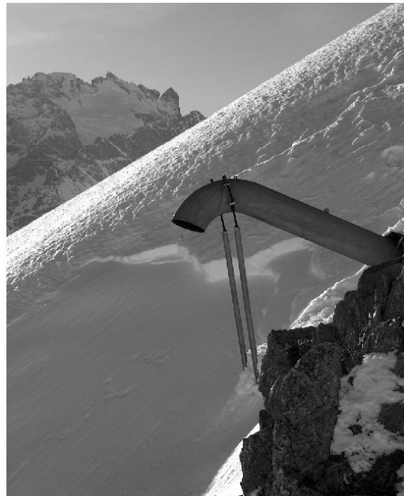
Figure 3. The release remote system GazEx used in avalanche path n°2.
