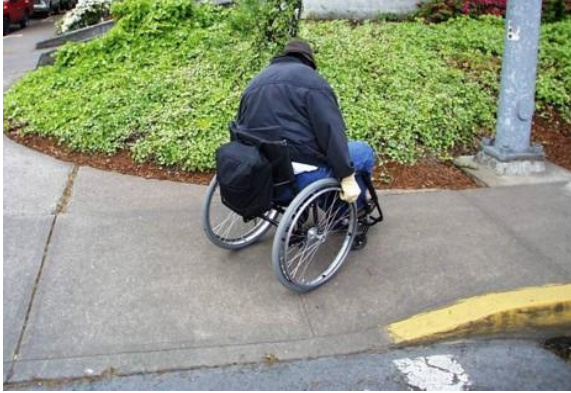
This is a bad example of a no top landing.
