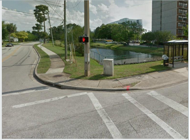
This is a bad example of no curb ramps at crossing.
