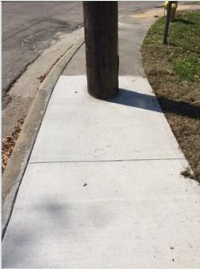
This picture shows a pole in the middle of a sidewalk, which is an accessibility issue.
