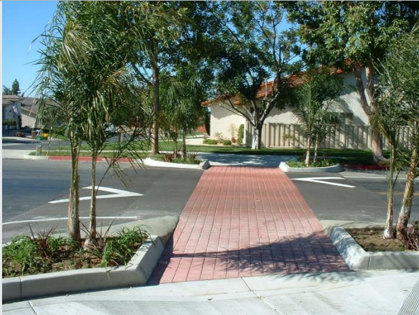
This is a good example of a raised crossing.
