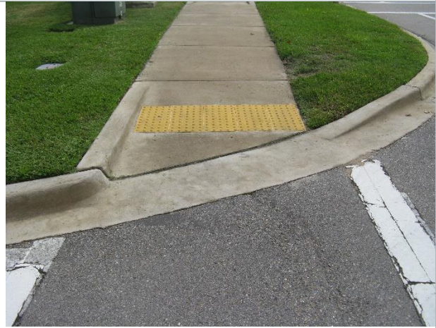
This is another good example of a detectable warning.
