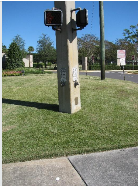
This is a bad example of an out of reach pedestrian pushbuttons.
