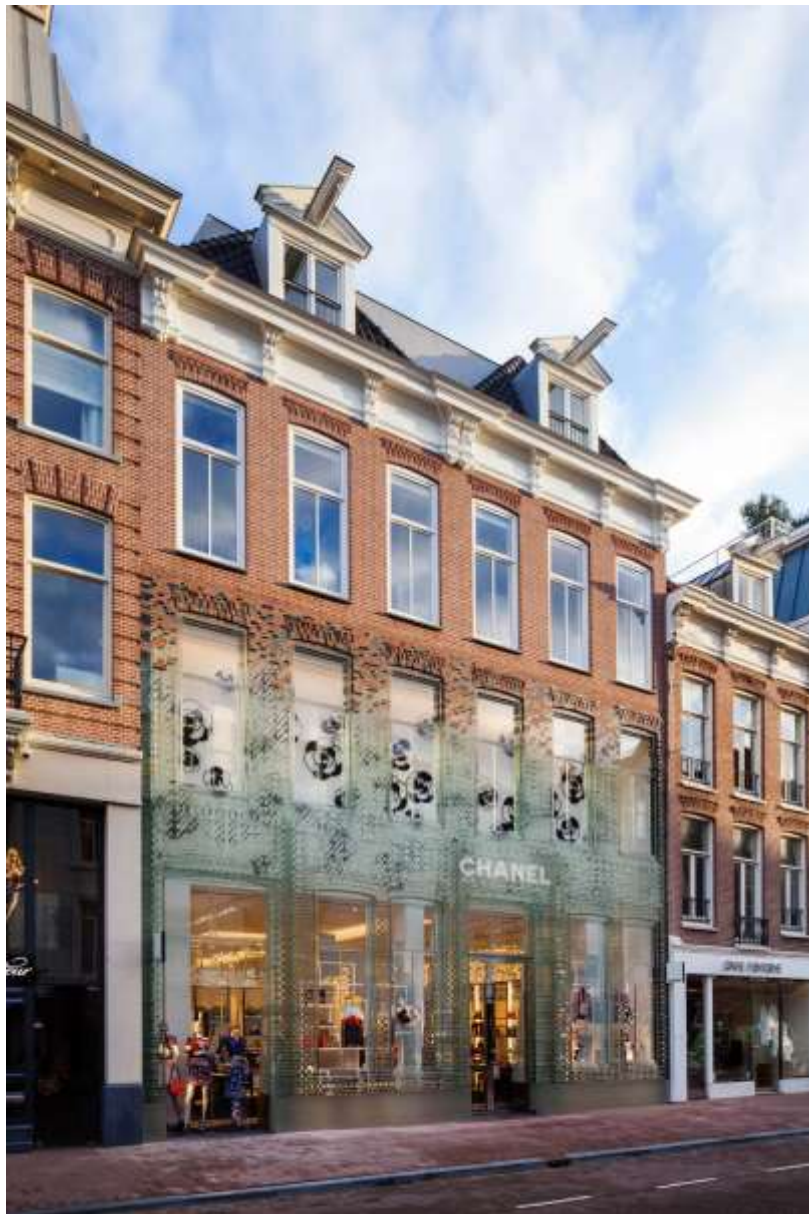
Gambar 8.11. Crystal House of Chanel di Amsterdam dengan fasad glass-brick . (Sumber https://www.archdaily.com dan https://www.yellowtrace.com.au/mrdv-crystal-facade-chanel-amsterdam-flagship/ )
