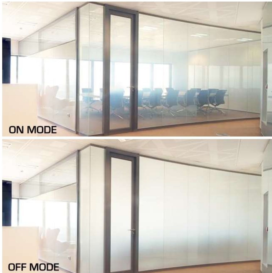
Gambar 2.36. Tampilan smart glass saat diaktifkan ( on-mode ) dan dinon-aktifkan ( off-mode ). (Sumber https://www.sgglassmanufacturer.com/products/Smart-Glass.htm )
