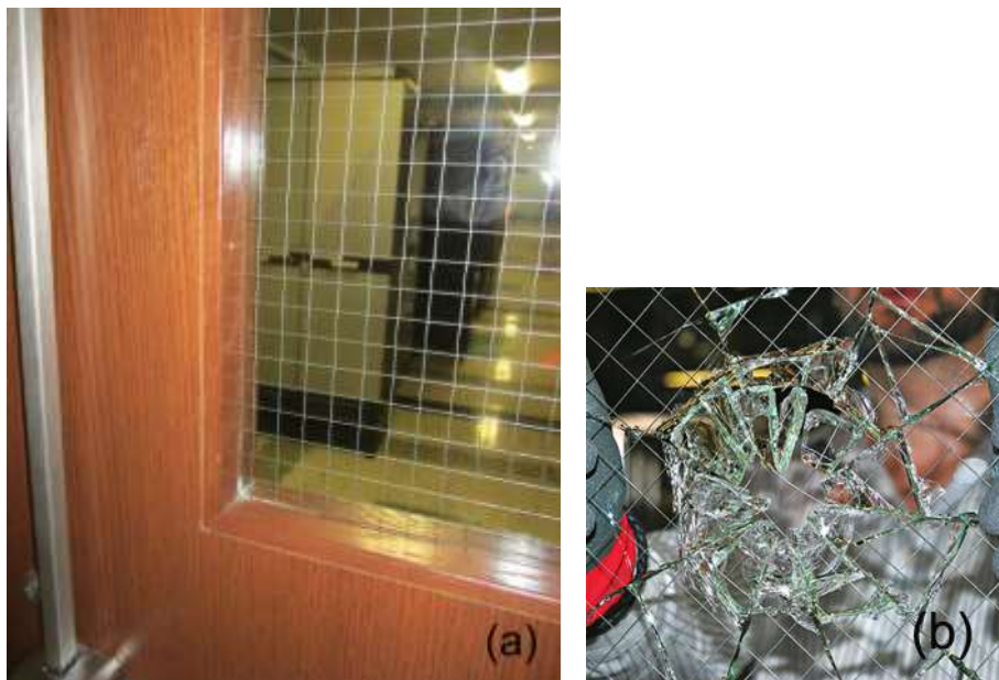
Gambar 2.43. Wired glass untuk pengisi daun pintu (a) dan keadaannya ketika pecah (b). (Sumber http://idighardware.com/2013/01/addressing-the-hazards-of-traditional-wired-glass/ dan https://www.constructioncanada.net/rethinking-wired-glass/ )
