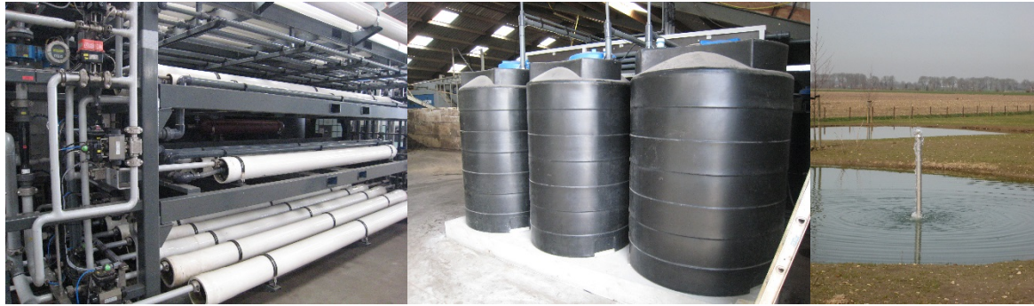
Photo 6.3. From suspended particles cleaned liquid passes the RO unit (left) which leads to mineral concentrate (middle) and clean water which can be discharged on surface water (right).
