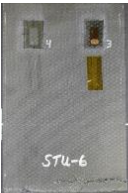
a) Back surface damage
