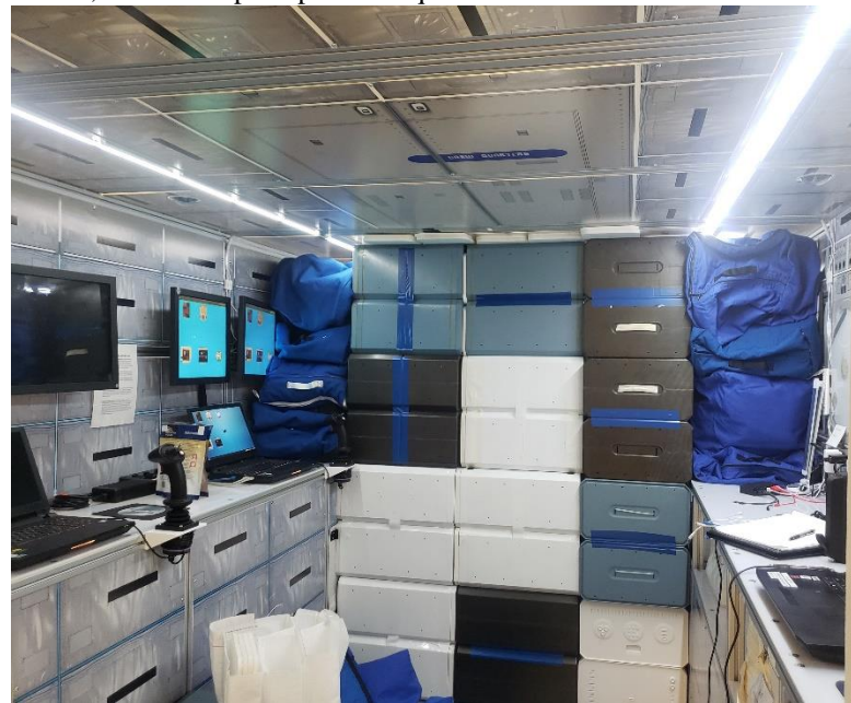
Figure 2. (Image Credit: NASA) Constructed rear wall of storm shelter in JSC habitat.
