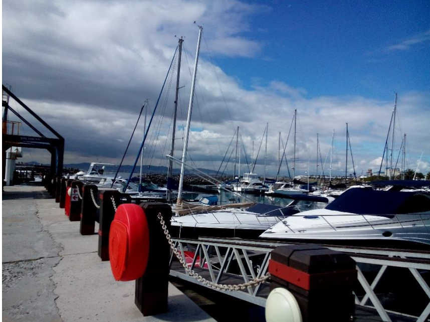
Figure A 1: Granger Bay Harbour (GRB)
