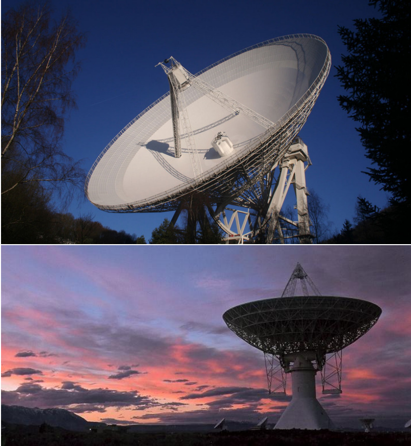
Figure 1.2: Top: The 100-m radio telescope in Effelsberg, Germany. Built in 1969, it is the second largest free steerable radio telescope in the world. Source: http://www.mpifr-bonn.mpg.de/337419/gallery_zoom.jpg Bottom: Owens Valley Radio Observatory (OVRO) 40-m dish. Source: https://www.ovro.caltech.edu/images/40m_small_4.jpg Data from both instruments, along with the Green Bank Interferometer (GBI), have been used for the thesis.
