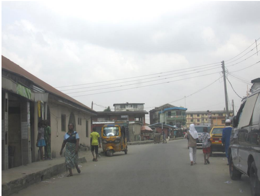
Figure 2.6: New road in Itire Slum, 2016 Constructed by Lagos state Government under the LMDGP
