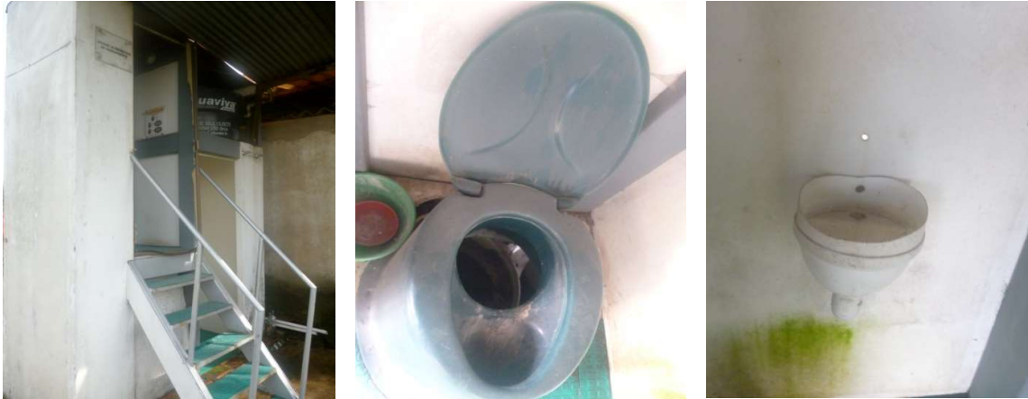
Figure 2.5. View of toilet closure.
