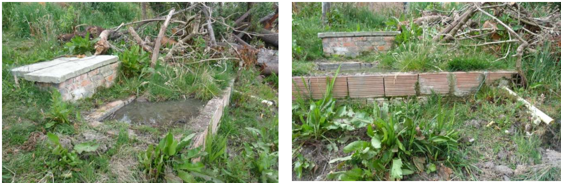
Figure 2.4. View of biofilter.
