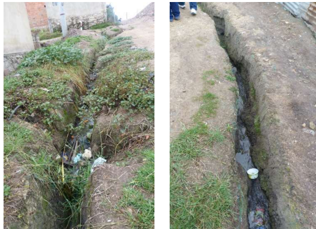
Figure 2.8. Rain water and wastewaters flow down the hill in the absence of sewage systems.
