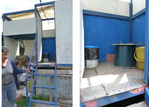
Figure 2.9. View of toilet closure in Ciudad Bolivar.
