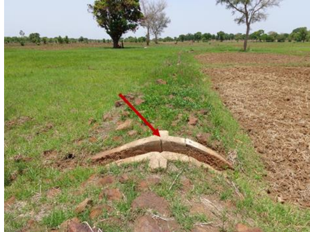
Fig. 2-7. Concrete flume (showed by the red arrow) for field water management in the Bankandi-Loffing catchment.
