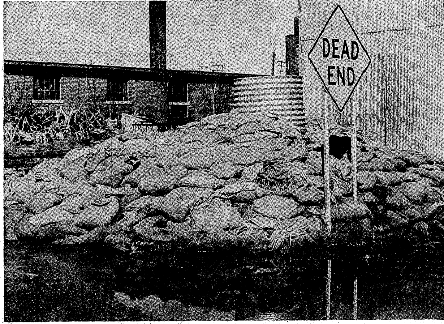
SIGN OF THE TIMES . . . A sandbag-reinforced sand-boil chimney blocks a roadway in the Kansas-Front Street area. Such structures now dot the area behind dikes as flood
