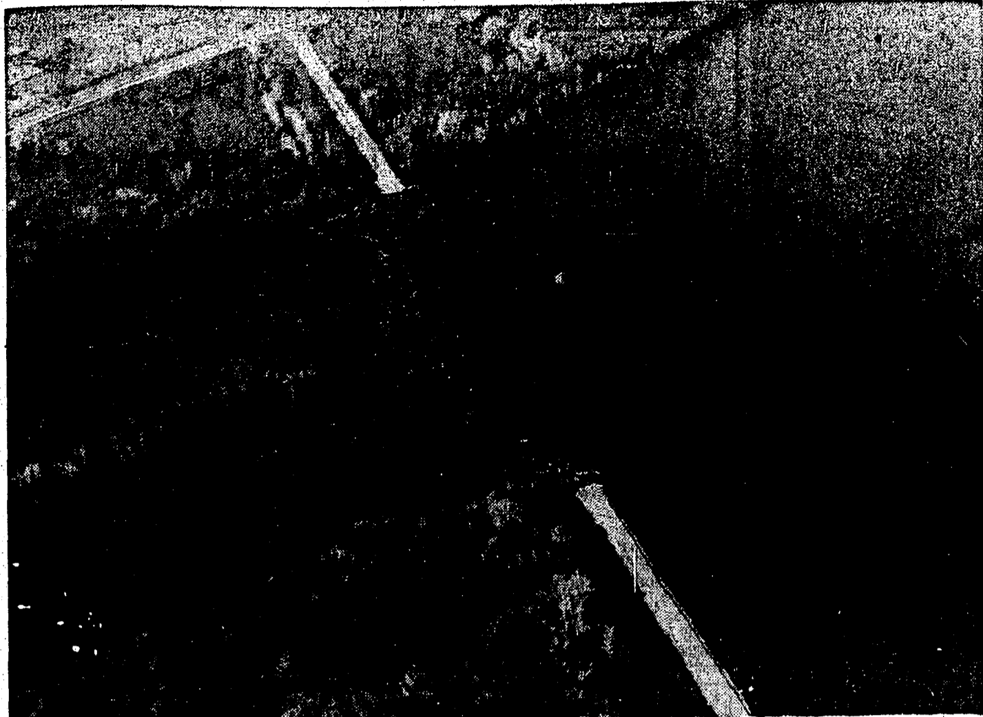
INUNDATED SPILLWAY . . . Looking toward Prairie Island Road in this aerial photo the turbulent water of the Mississippi River is rushing to the left over the concrete Prairie Island spillway, center, an area of 1,000 feet, on the west side of Winona. The spillway, which is part of Winona Lock & Dam 5A, extends into Wisconsin. Wally Voss, lockmaster at
