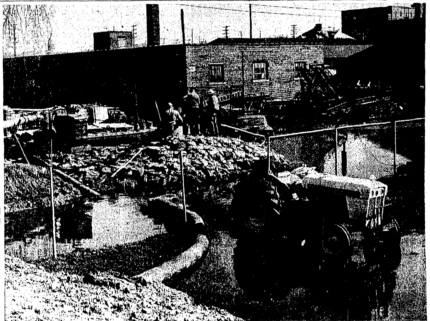
LITTLE DANDY . . . Pumps like this one are credited by City Engineer Robert J. Bollant with doing yeoman service in the present flood situation. Designed originally for irrigation work by a Montana manufacturer, the pump operates under water with power furnished by whatever source is
