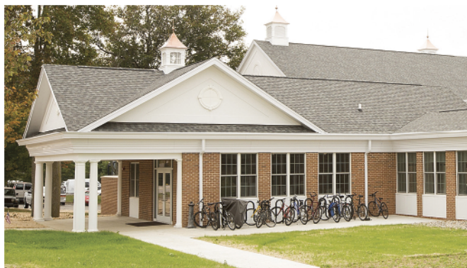
Exterior renovations to Simpson Residence include a new covered entry and a hip roof.
