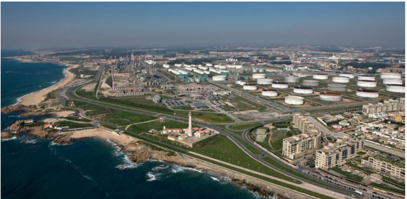
Figure 2.5: Matosinhos refinery - Galp Energia S.A. (Galp Energia, 2010b).
