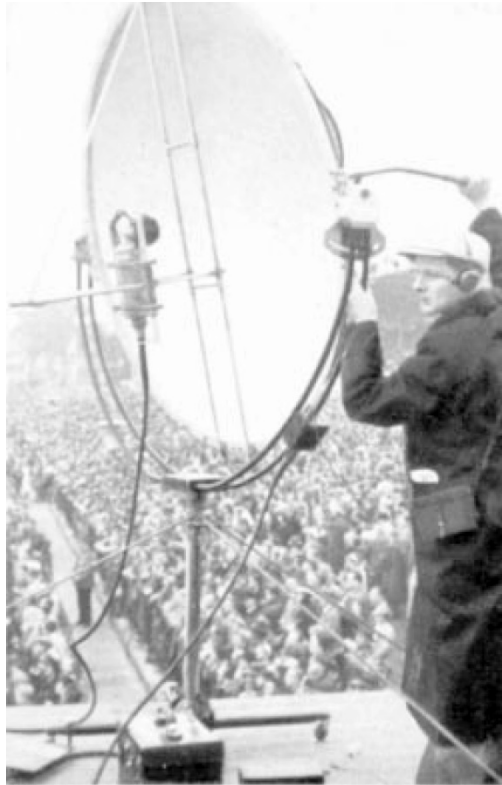
Figure 10 : A parabolic microphone used in the 1936 Olympics for capturing rowing and sailing
