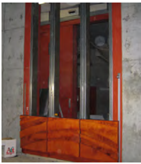
Figure 46: Construction of test sample
