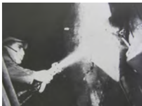
Figure 16: Application of asbestos sound absorption
