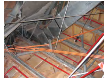
Figure 35: Concert Hall ceiling construction
