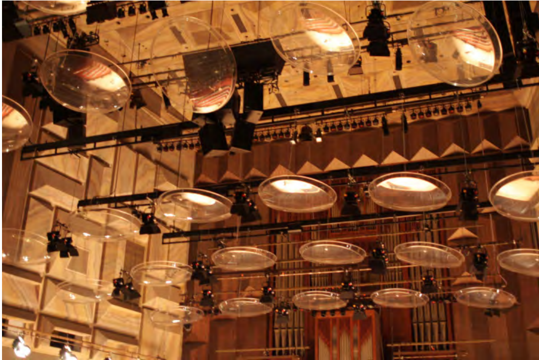
Figure 43: Melbourne Concert Hall above stage reflector array (prior to renovation)
