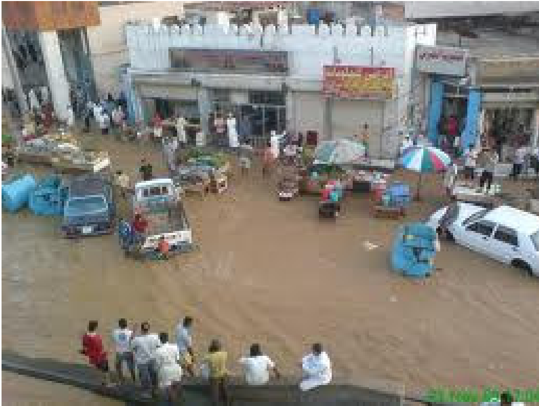
Picture 2.4: The lack of a drainage network, which affects the city almost every year in the rainy season
