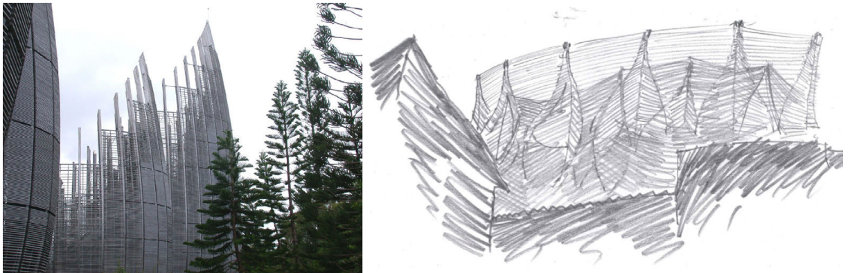
Figure 4.7: The design of permeable structures to interact with the wind flow, in a more sophisticated way, is a current field of exploration by architects, that requires working with wind analysis tools in the early design stage. Left: Jean Marie Tjibaou Cultural Center, designed by Renzo Piano, 1998 (taken from Waters 2003 CC BY-NC-ND 2.0). Right: Windshape pavilion by nARCHITECTS, 2006 (Author's sketch based on ( Arch-Daily 2008 )).
