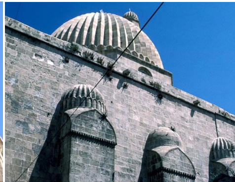
Figure 37. The Great Mosque from the southwest showing ribbed domes of the minaret, sanctuary dome and qibla wall buttresses, Mardin, 1984. 337
