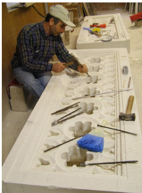
Figure 27. Stonemason Ramazan Güduloğlu finishing ornamental tracery of a balustrade for Dolmabahçe Palace, Istanbul, 2007. 277
