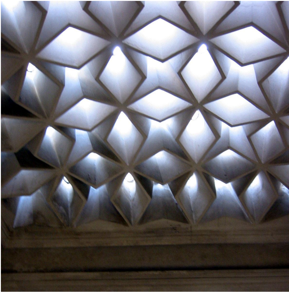
Figure 1. Bathroom ceiling from Dolmabahçe Palace, Istanbul, 2006. 28
