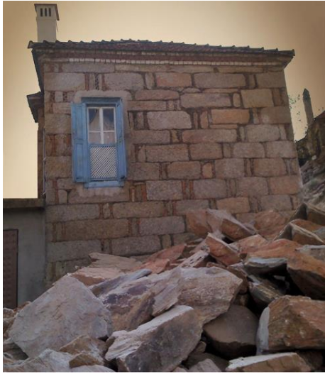
Figure 60. House from Çomakdağ, an inland Aegean mountain village, with stones piled up in front to build an extension, 2011. 483
