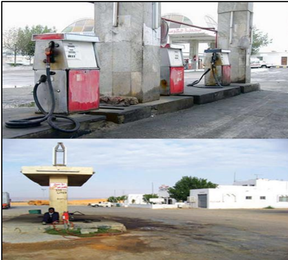
Figure 5.7: Petrol leaks issues in Saudi Arabian petrol stations
