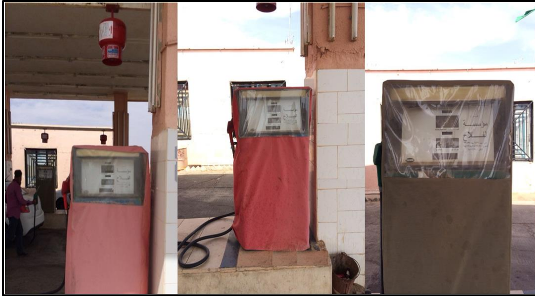
Figure 5.6: Petrol dispensers are covered due to the dust storms and extreme heat in Saudi Arabia
