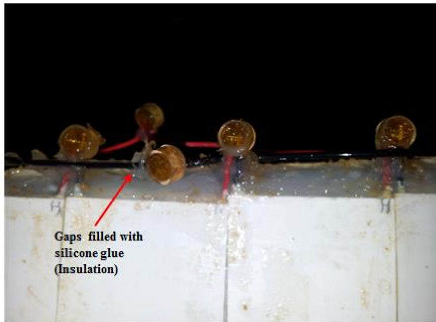
Figure 5.21 Insulation of the gap using silicone glue
