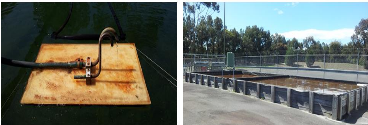
Figure 3.22 Flushing system (left) and evaporation ponds at RMIT University solar pond.
