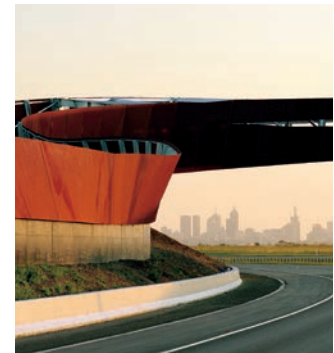
Above: Craigieburn Bypass, a Sticky Project, which was the first large infrastructure project TCL had undertaken.
