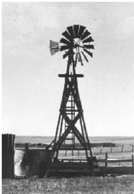
Figure 2.1: Steel-bladed water pumping windmill in American Midwest in late 1800s (Image courtesy: http://telosnet.com/wind/early.html )
