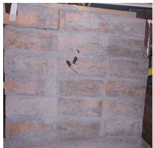
b) Exterior brick wall (outside view)
