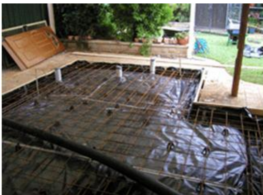
a) H-class reinforced concrete slab
