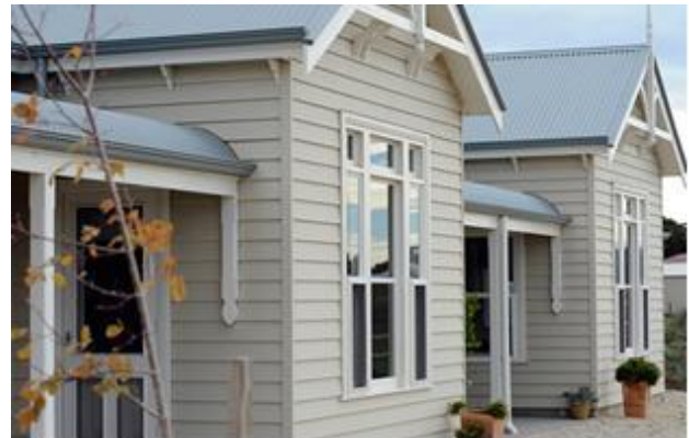
b) Typical timber weatherboard house
