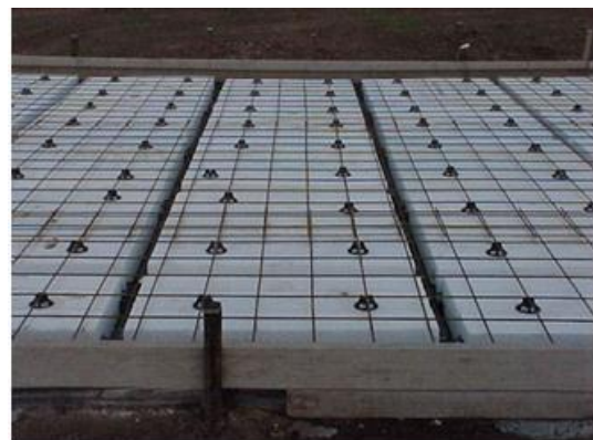
b) Waffle concrete foundation
