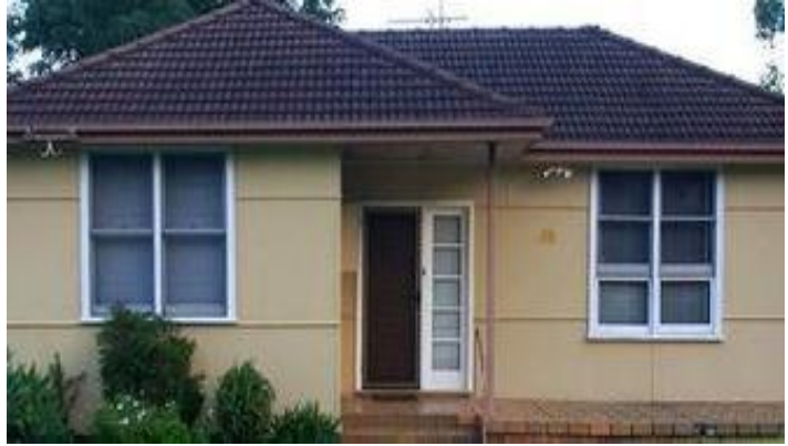
b) Typical fibro cement weatherboard house
