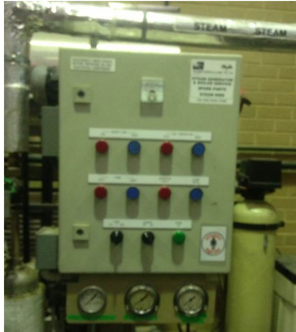
Figure 7-4 Pressure controller
