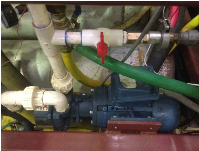
Figure 7-48 Vacuum pump
