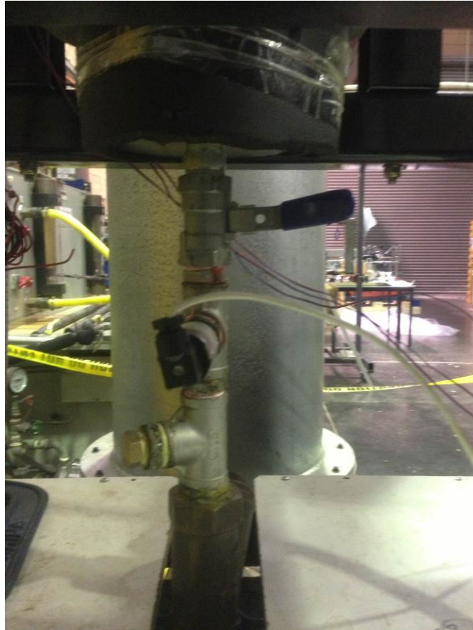
Figure 7-50 Inlet hot water valve to vacuum chamber
